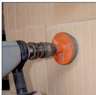
Mark around the socket outlet and drill a round hole using a commercially available drill and dry diamond core drill bit.
