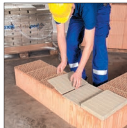
Lay on Maxit mortar pads
