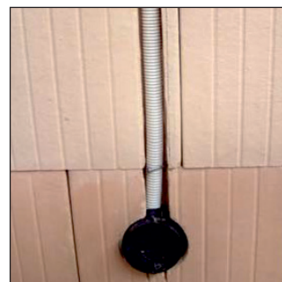
Insert the electrical installation into the slot.
