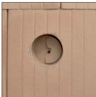
Remove any JUWO POROTON Block remains and drilling debris – and insert the socket outlet.
