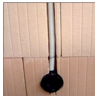
Insert the electrical installation into the slot.
