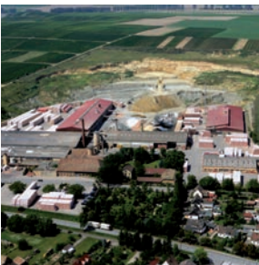
Aerial view of JUWO company site (Headquarter Wöllstein)
