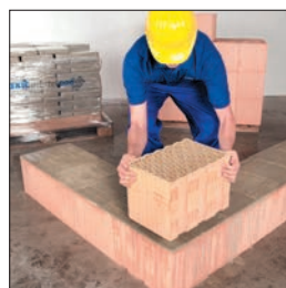
Lay blocks with full surface
