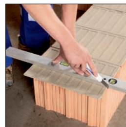
Cut and adjust Maxit mortar pads if necessary
