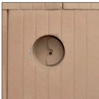
Remove any JUWO POROTON Block remains and drilling debris – and insert the socket outlet.
