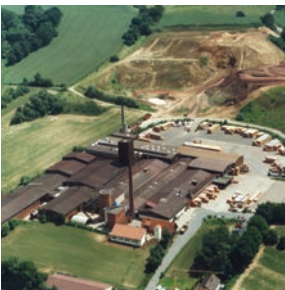
Aerial view of JUWO location Zeller Poroton, Alzenau (Bavaria)
