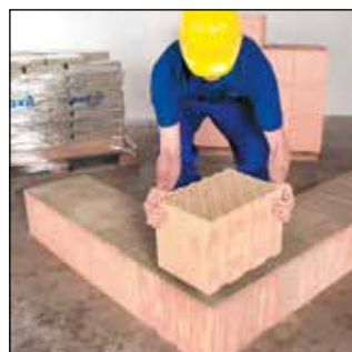
Lay the brick over the entire surface
