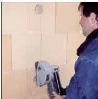
Slot the bricks with the slot cutter.
