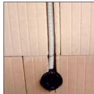
Inserting the electrical installation into the slots.
