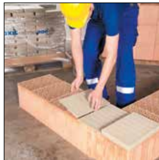
Lay on maxit mortar pads
