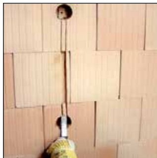
Knock out the pre-sawn slots with a hammer and chisel.
