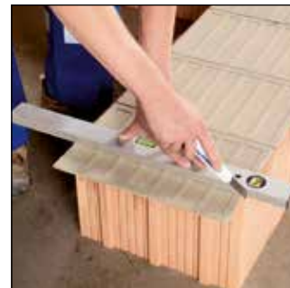
Cut maxit mortar pads to size if necessary
