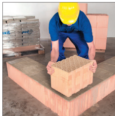
Lay blocks with full surface
