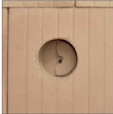
Remove any SmartWall Block remains and drilling debris – and insert the socket outlet
