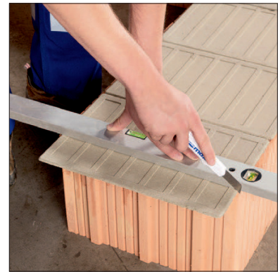
Cut and adjust Maxit mortar pads of necessary
