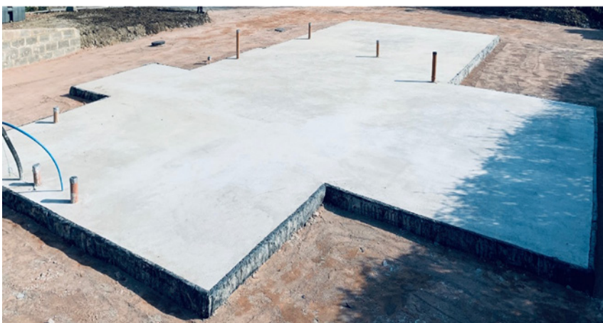
SmartWall Blocks placed on a DPC to complete the seal
