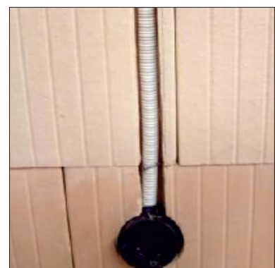
Insert the electrical installation into the slot
