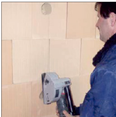
Use the wall chaser to cut slots in the SmartWall Blocks
