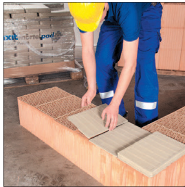
Lay on Maxit mortar pads
